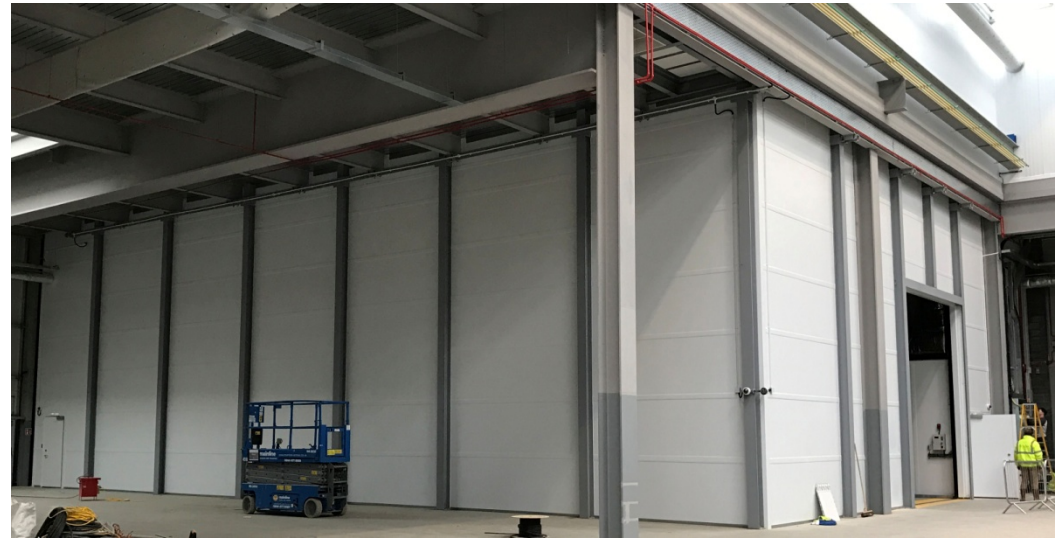
Horizontally fixed wall panels allow construction to any height (over 8m in this example). High security testing cell
