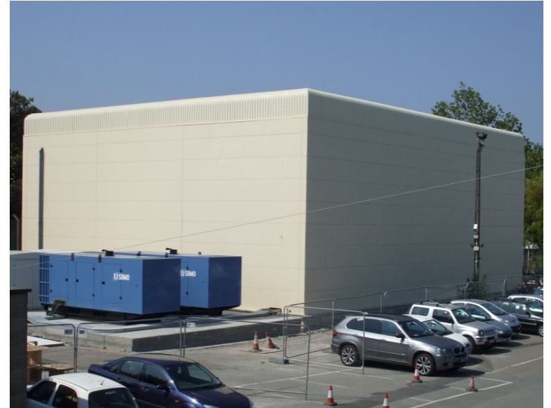
2 storey data centre plus flat roof deck for plant. External cladding.
