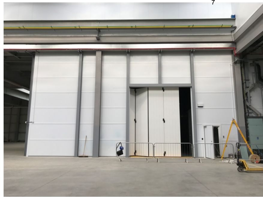
Horizontally fixed wall panels allow construction to any height (over 8m in this example). High security testing cell
