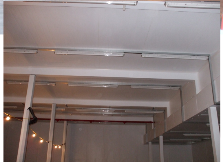
Smaller internal steels with shorter spans
