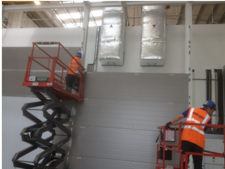
Horizontally fixed wall panels allow construction to any height (over 8m in this example). High security testing cell
