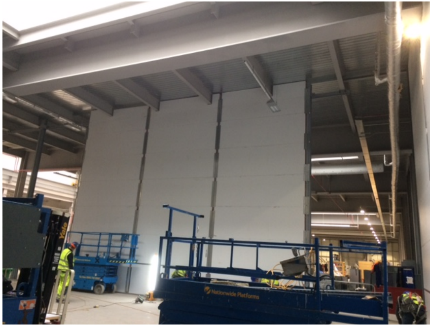
Horizontally fixed wall panels allow construction to any height (over 8m in this example). High security testing cell
